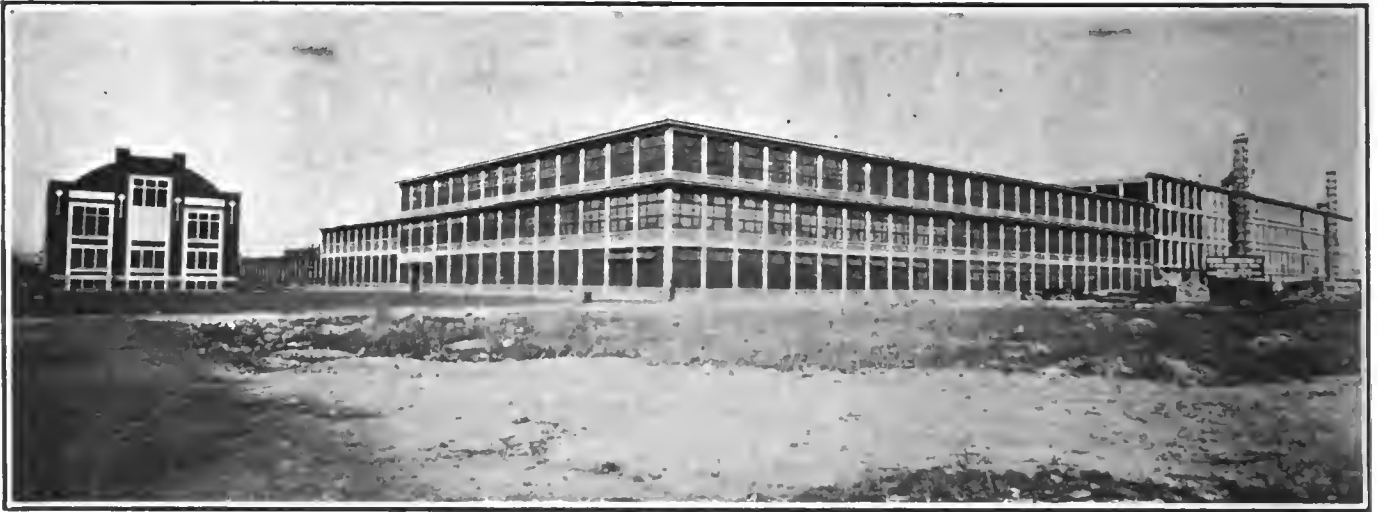
Panorama view of the Pierce-Arrow plant along Great Arrow avenue. The three-story structure in the foreground is one wing of the original body building, while at the right may be seen one of the four-story 350 by 60 foot wings just added to it. At the left is shown one end of the Administration building.
